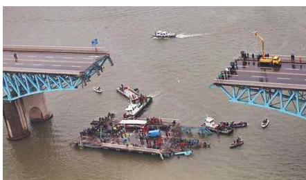
<Failure of Sungsu bridge, 1994>
