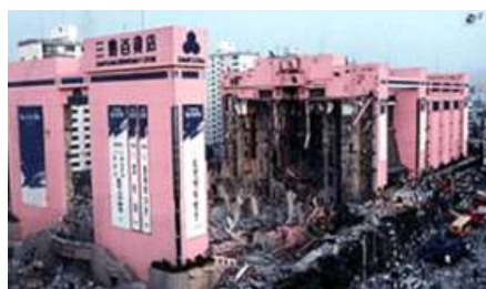
<Failure of Samping department store, 1995>
