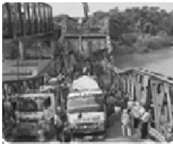
Cipunegara Bridge July 23, 2004 Collapsed because of overloading
